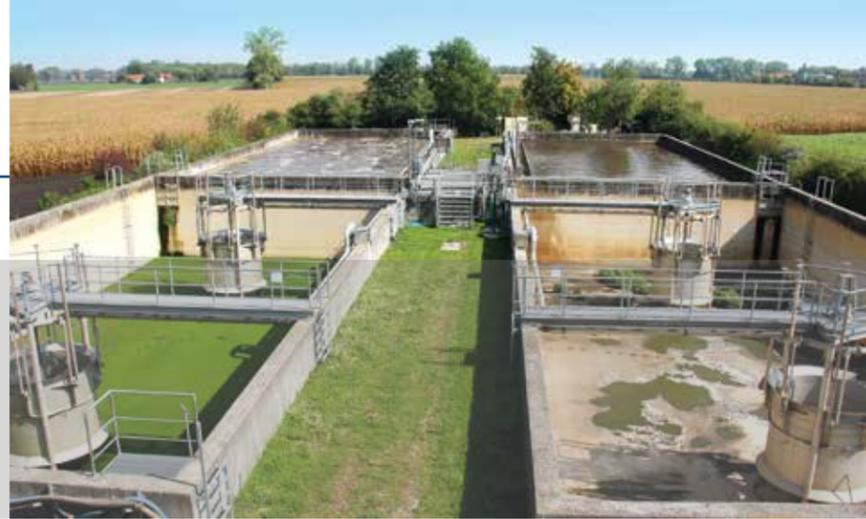
At the Oberschleißheim wastewater treatment plant, as part of the energy optimisation measures, two of the four aeration tanks were taken out of operation.
