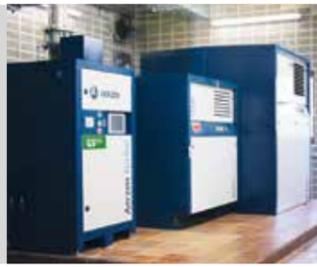
In the wastewater treatment plant at Oberschleißheim, the AERZEN Performance³ technology mix consisting of a turbo, a Delta Blower and a hybrid machine ensures an efficient compressed air supply in the aeration tanks.
