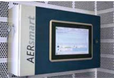
The AERZEN integrated control system AERsmart distributes the required volume flows to the machinery in such a way that low, medium and high loads are processed as efficiently as possible.
