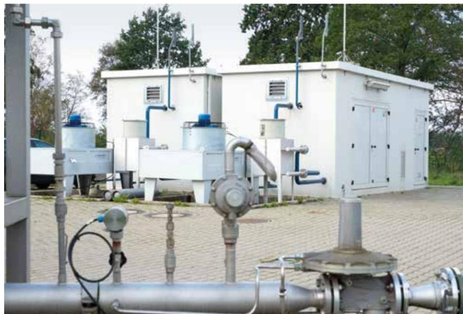
Each assembly delivers a flow rate of 700 standard cubic metres per hour - and is certified for this application in accordance with ATEX.
