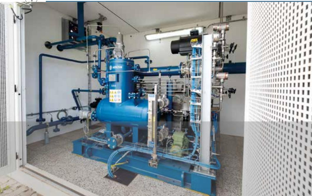
Screw compressors from AERZEN compress the biomethane for feeding into the local gas network.
