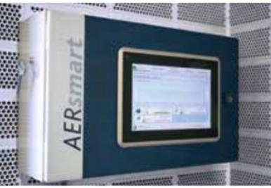
The AERZEN integrated control system AERsmart distributes the required volume flows to the machinery in such a way that low, medium and high loads are processed as efficiently as possible.
