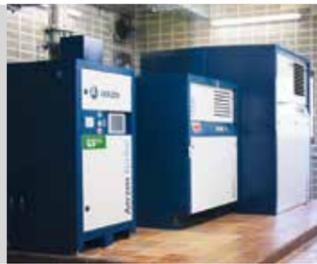
In the wastewater treatment plant at Oberschleißheim, the AERZEN Performance<sup>3</sup> technology mix consisting of a turbo, a Delta Blower and a hybrid machine ensures an efficient compressed air supply in the aeration tanks.
