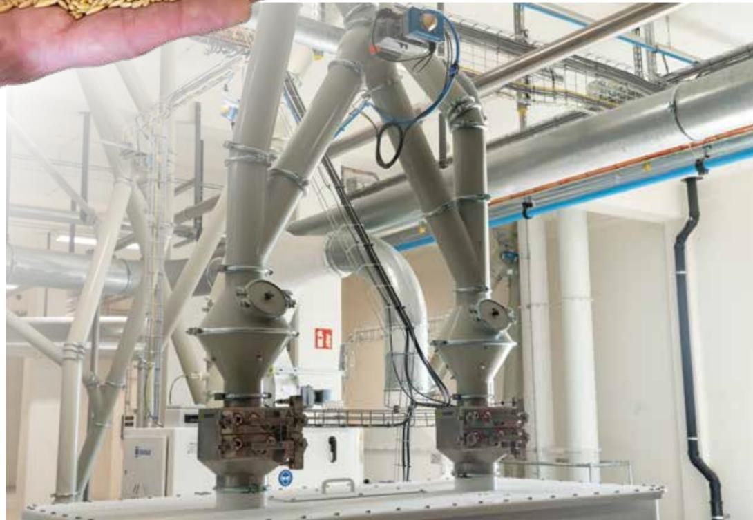
The Delta Blowers take over the pneumatic transport of the grain kernels, intermediate products and finished flakes.
