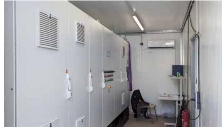
The control system for the turbo blowers is housed in a separate container. As the technology of the wastewater treatment plant was destroyed by the flood, the control of the mobile rental solution runs separately.
