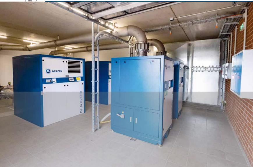
The combination of turbo blower and rotary lobe compressor creates the basis to cover the oxygen demand in the activation with maximum efficiency.
