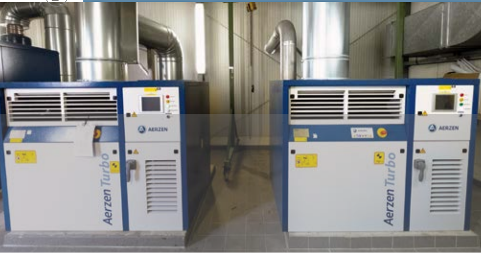
The two turbo blowers from AERZEN cover the basic load of the wastewater treatment plant. Each turbo blower delivers up to 5000 standard cubic metres.
