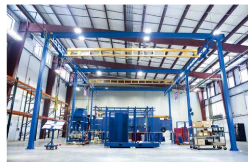
The new Turbo Blower assembly line
