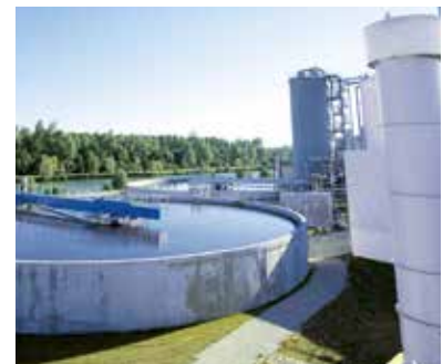
Efficient aeration in sewage plants: made possible by AERZEN technology
