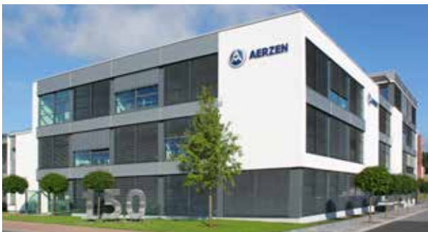
Opened in 2013/14: the new administration building in our home town of Aerzen
